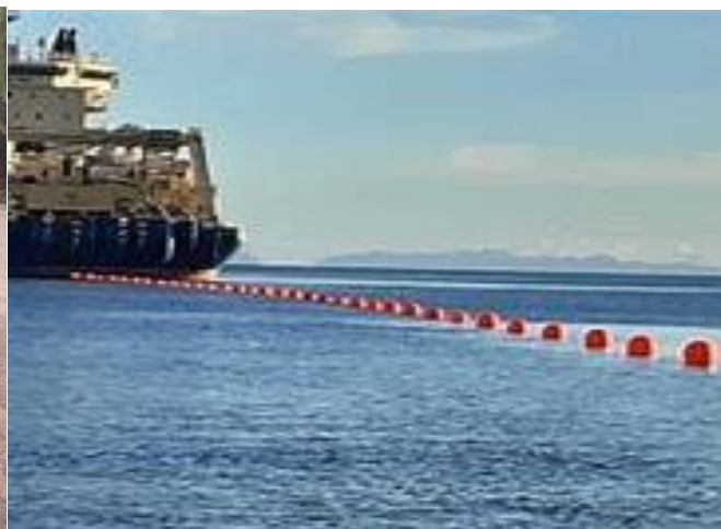
Fig 17: Cable laying with the boat offshore
