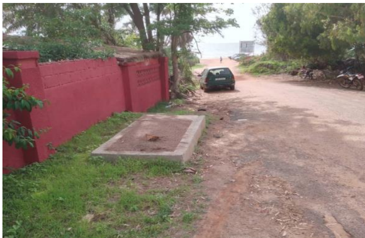
Fig 16: Beach ManHole of the ACE Cable
