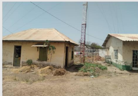
GAMTEL exchange station at Kuntaur, CRR
