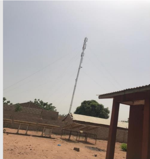
GAMTEL exchange station at Njaba Kunda, NBR
